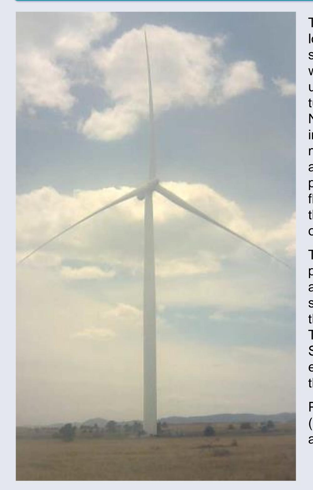
This measurement campaign looked into measuring vortex shedding on a flatback airfoil of a wind turbine blade through the use of a highly-instrumented test turbine (SWT-2.3-108) at the National Wind Technology Center Boulder, CO. Pressure IN made measurements were around the flatback airfoil, with a particular interest in the pressure fluctuations on the trailing edge of the airfoil, where vortex shedding occurs.
