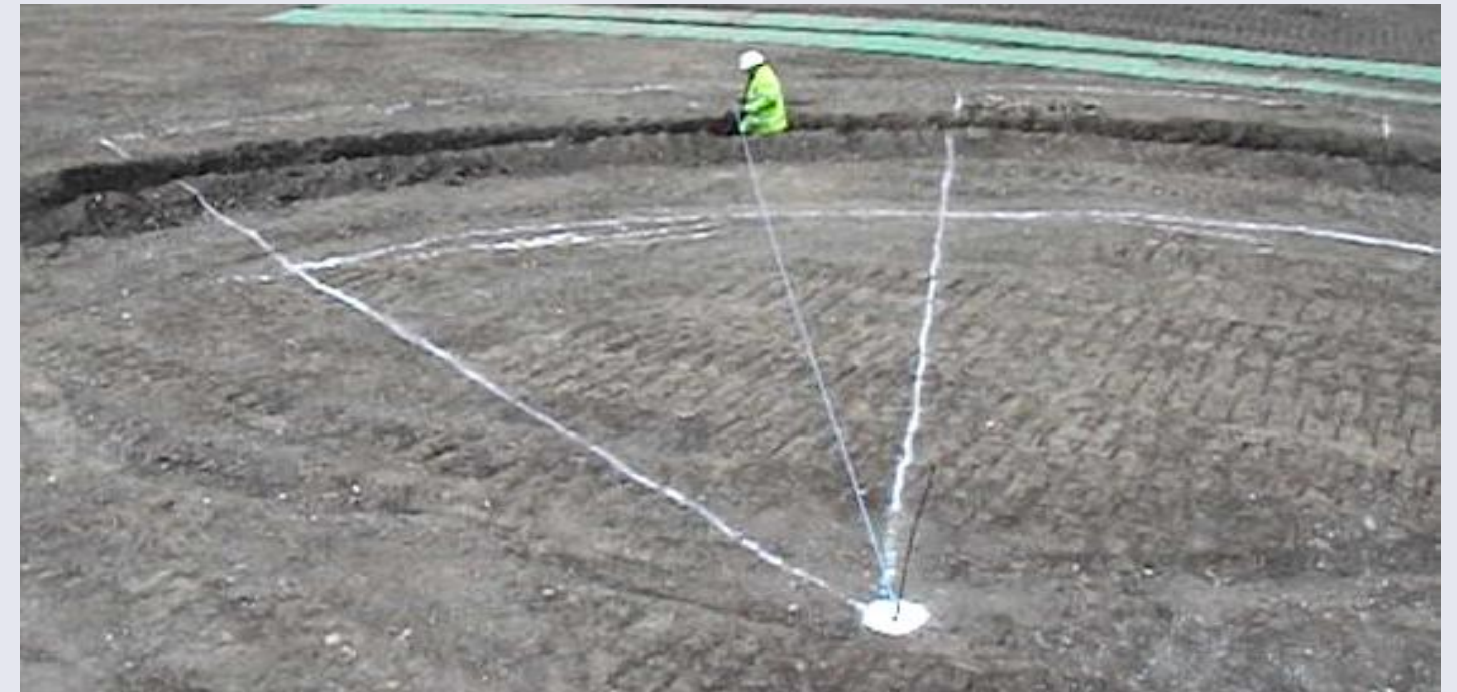
Figure 3. Demonstration of tight turning radius for trenching vehicle
