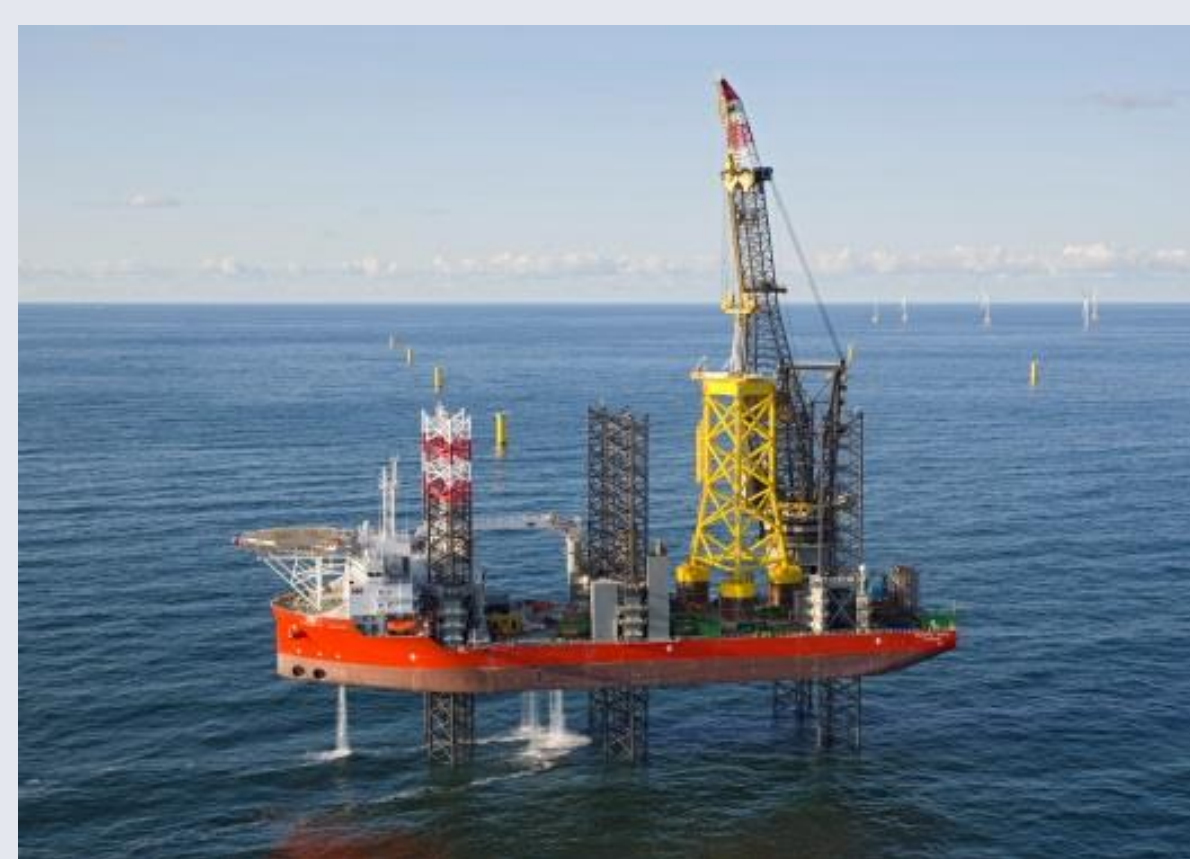
Installation of BKR01 suction bucket jacket foundation, August 2014
