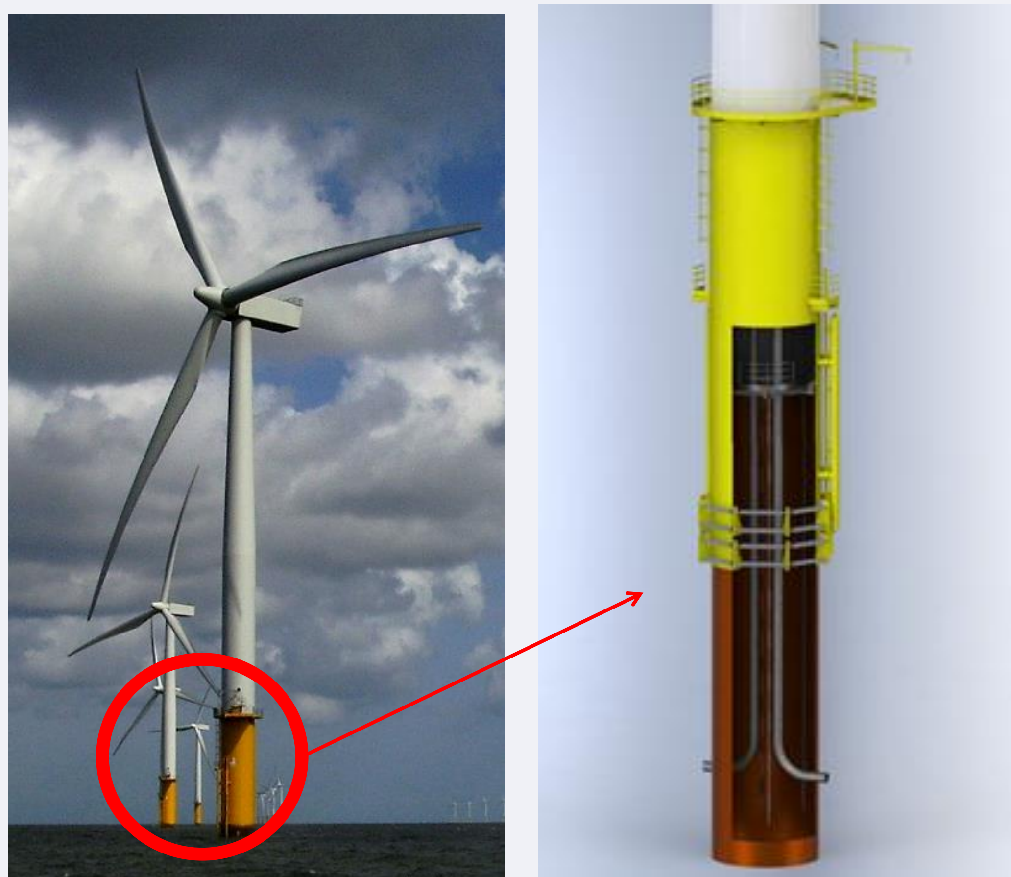
Figure 1 – General arrangement of monopile foundations
