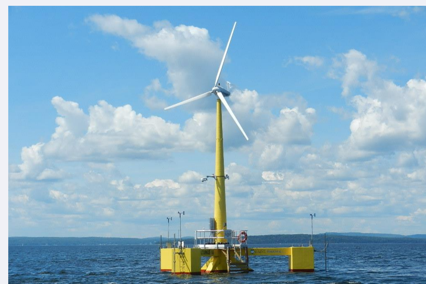
VoltturnUS 1:8 installed off Castine, Maine, USA
