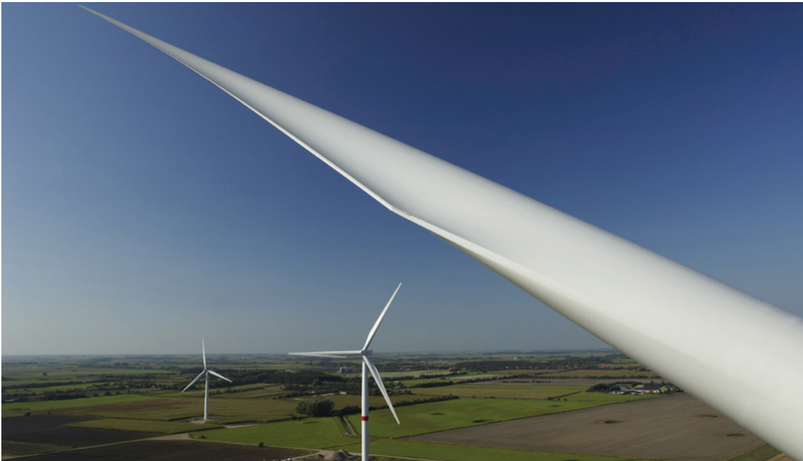
Photo: Siemens AG Energy Sector
