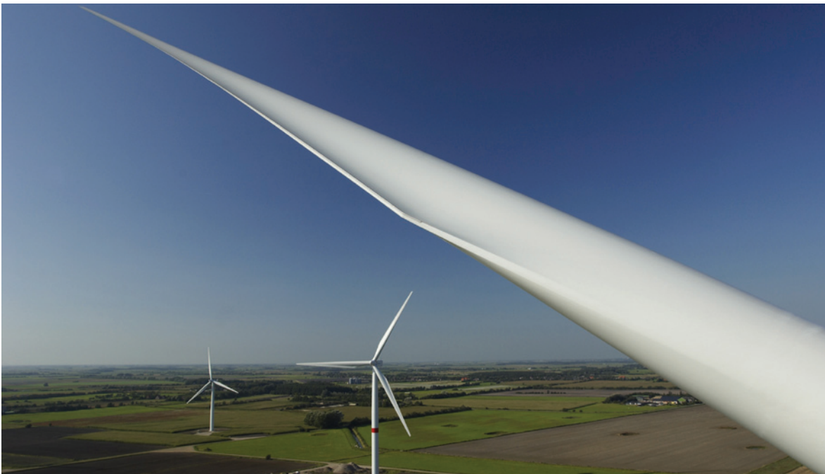
Photo: Siemens AG Energy Sector
