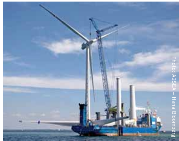
Leg-stabilised crane vessel A2Sea Sea Power at Lilligrund
