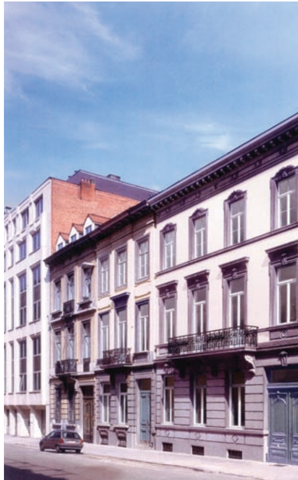
EWEA's offices are located in the Renewable Energy House in the centre of the European quarter of Brussels
