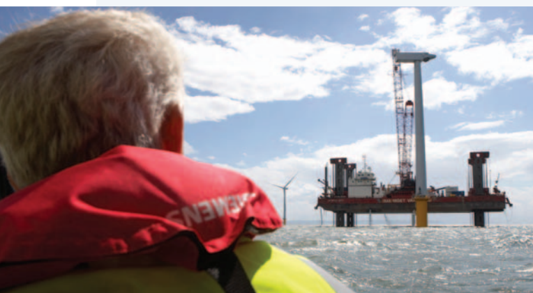
Burbo Bank wind farm, UK (© Siemens AG)
