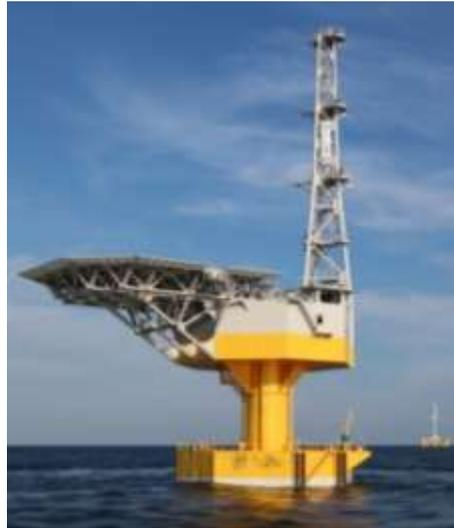
Figure 1 The substation of the Fukushima Floating Offshore Wind Farm
