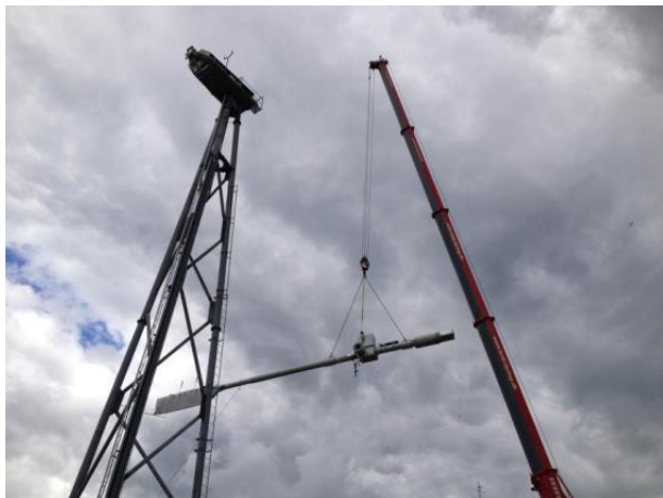
Figure 4 The photo to the left shows installation of the boom with the blade section in June 2014. On the photo to the right the blade section with the flap (black colour) can be seen as well as the two five hole pitot tubes.
