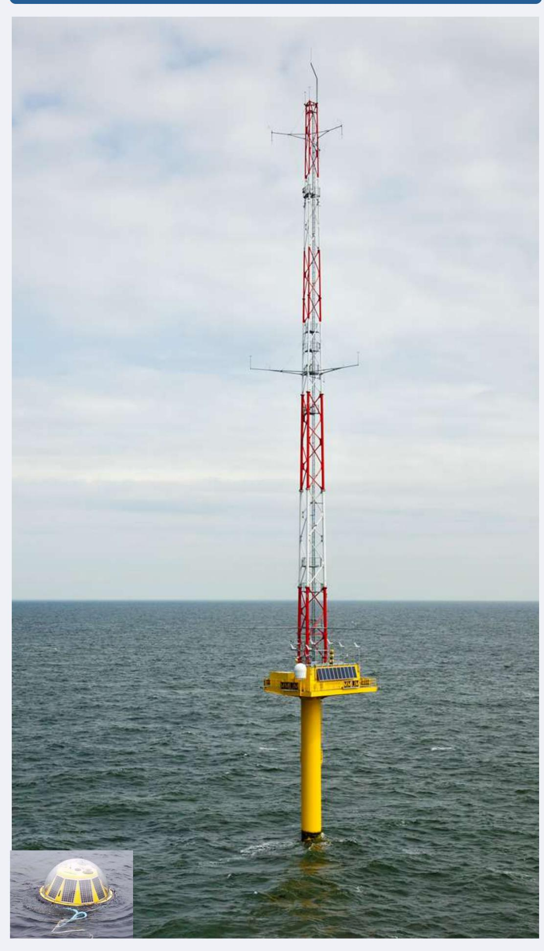
The current facilities comprises of a meteorological mast which is located approx. 75 km out of the coast of the Netherlands. The mast of 92m (AMSL) is owned by RWE and operated by ECN. At three heights (26, 58 and 84m) booms are placed for performing standard meteorological measurements. Besides these measurements also met.ocean data is collected with a buoy and a fixed LiDAR is placed on the platform. Furthermore on Lichteiland Goeree (a fixed platform) data is collected with a fixed LiDAR)
