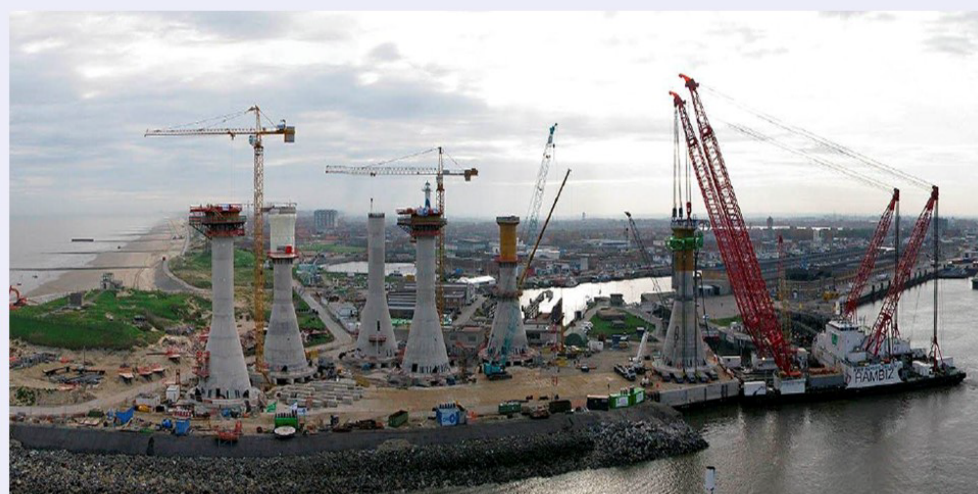
Figure 2: GBF construction at port of Oostende [5]
